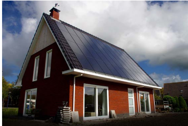
Netherlands, Friesland New family home installed by Friesland Solar
