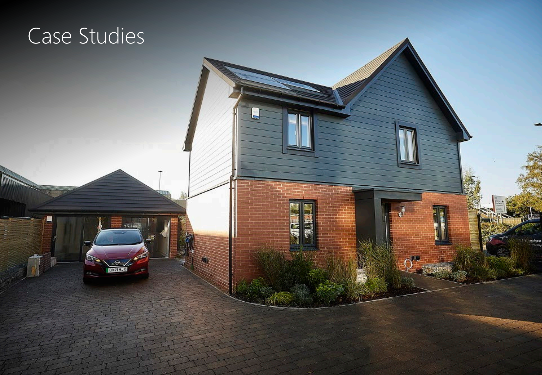
Salford, UK Barratt 'Z House' Zero carbon operational house
